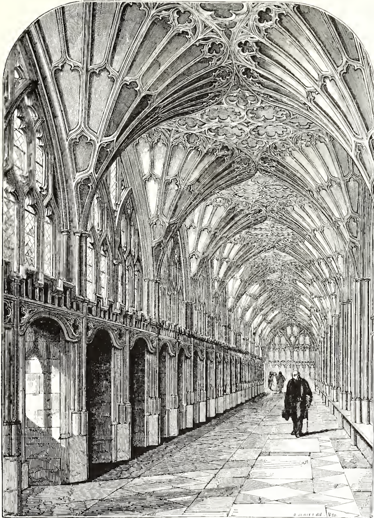
Fig. 54. View of the scriptorium alley of the cloisters at Gloucester, showing the recesses to hold the wooden carrels for the scribes or readers of manuscripts.
